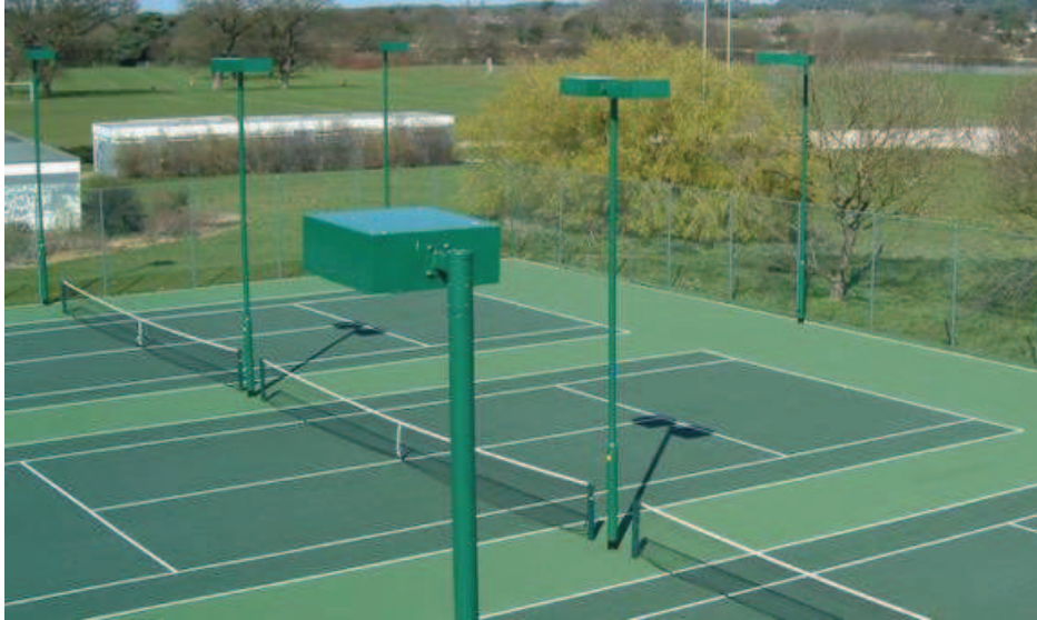
HI-LUX – Match107/WB 17B fittings installed on tennis courts with the type of columns proposed for Canons Leisure Centre
